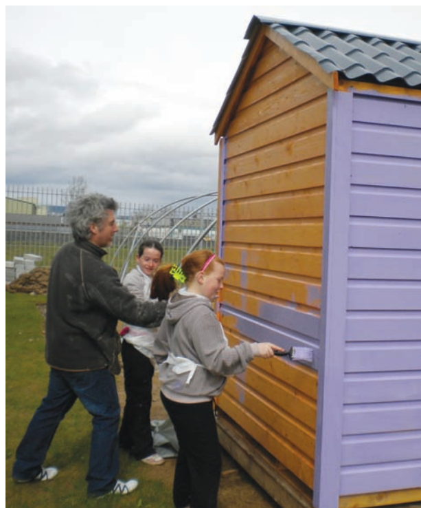
Constructive activities in Southill, Limerick
